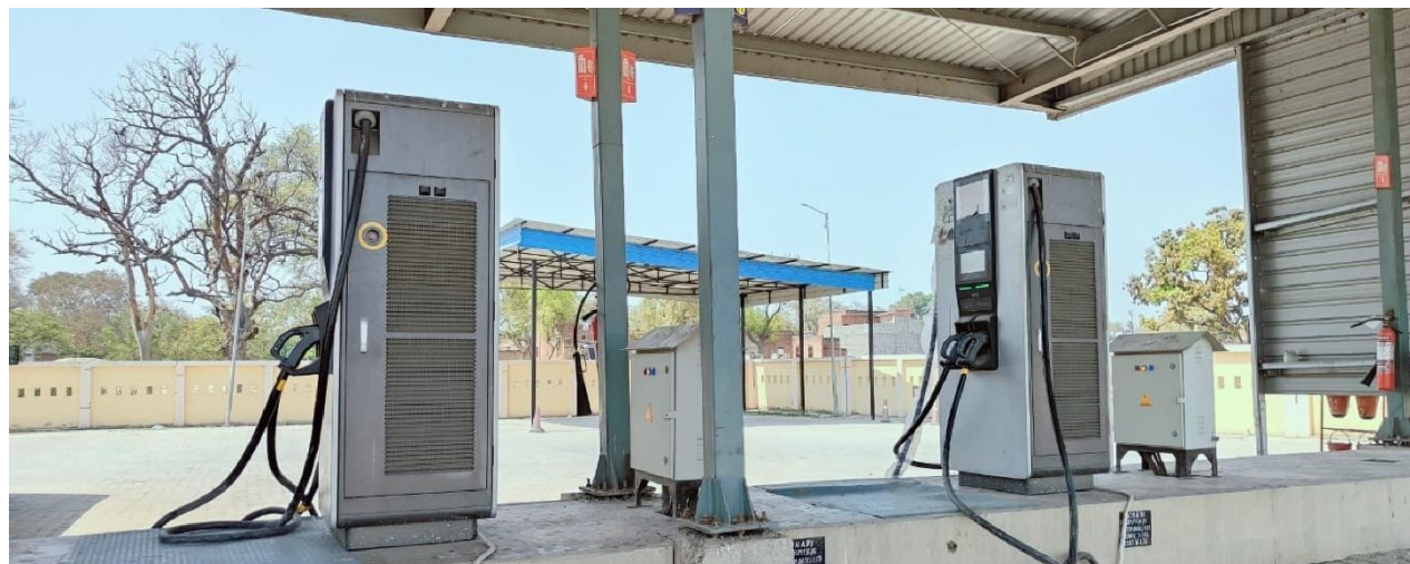
Figure 17: e-bus charging station at depot in Varanasi-3
